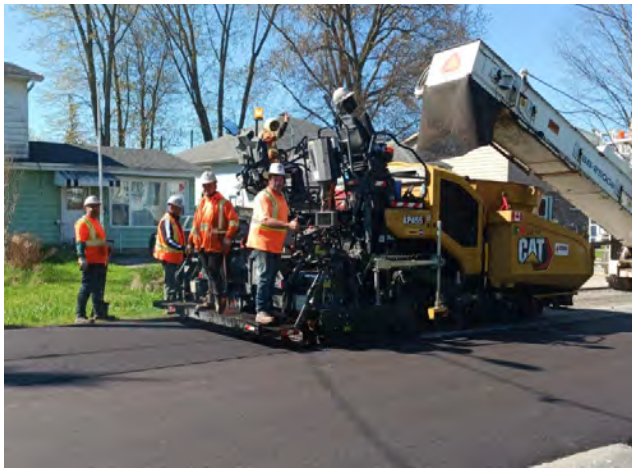
Figure 2: Resurfacing of Woodycrest Road – May 2025
