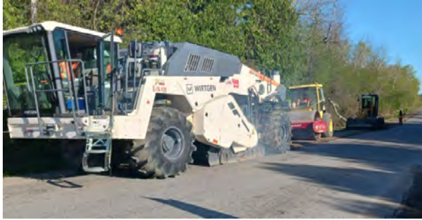
Figure 1: Resurfacing of Stoney Batter Road – May 2025
