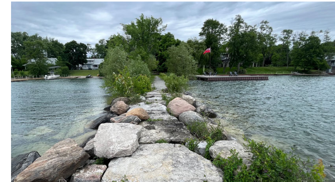
Raines Street/Roches Point Pier 2
